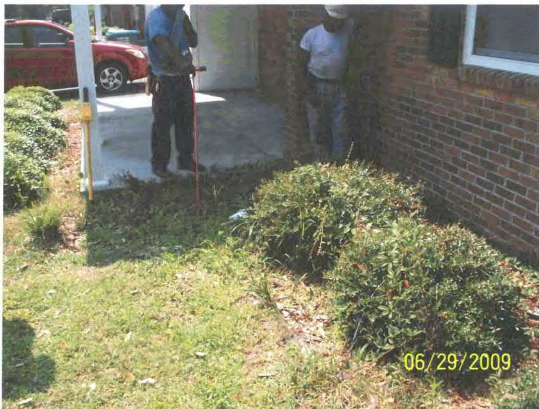
Picture 1: Location of UST 484Laurelbay prior to excavation.
